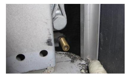
5) Once the tube is in place, simply add air with a bike pump, or air compressor. Very low pressure is all that is needed. You should be able to easily compress the seal with your hand. If it is overinflated it will feel hard to compress. The low pressure helps to seal around ice and debris.
