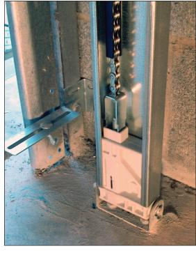
3. Stand the opener upright with the header bracket toward the floor.
